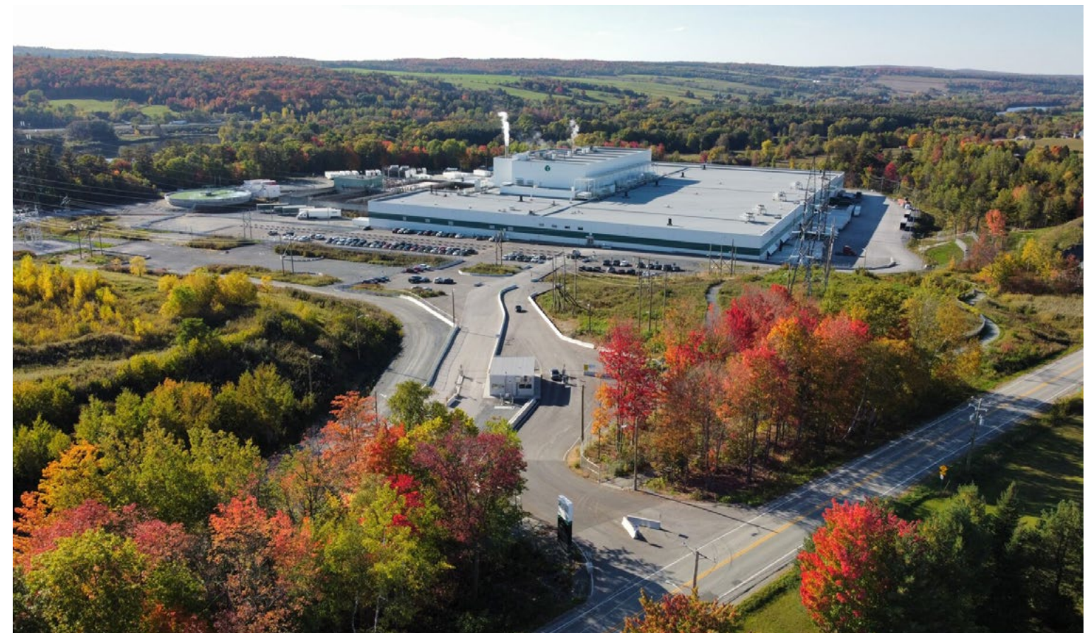
Sherbrooke, QC plant, commissioned in 2021
